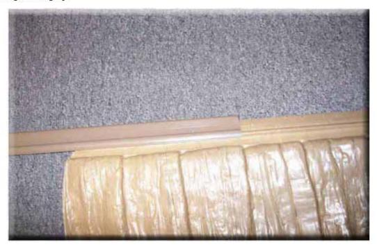
You then turn the leaf over so the fingers are sloping down. Now fold the rail over the thatch as shown in the above picture. Be sure some thatch is above the rail.
